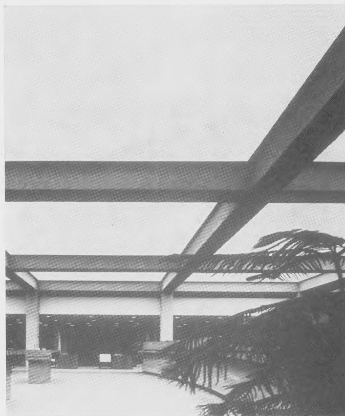
Illusion of expansiveness is created by lighted ceiling crisscrossed by massive wood-covered beams at First National, Lawrence, Kan.
