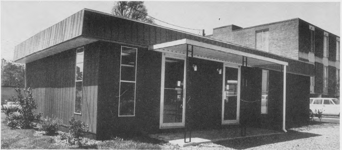
Virginia Capital Bank, Richmond, opened recently in this USRY-supplied modular unit that was towed to the site in two sections and bolted together on a permanent foundation. Four teller stations, a drive-up window and night depository are included.
