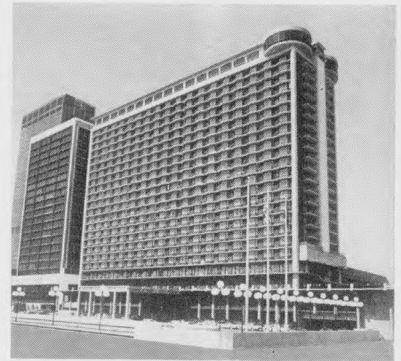
This is new Galt House in Louisville, headquarters for KBA's 1973 convention. At top right is twin-revolving penthouse restaurant with 20-mile views.
