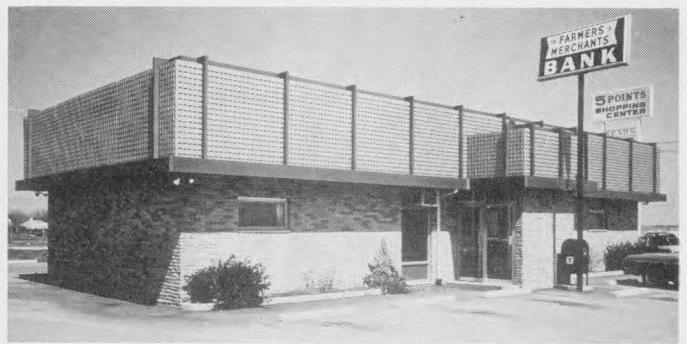
AFTER —Is this the same bank? Everything is the same except the "facia-wal" architectural paneling applied to square off the roof line. Now it looks like a bank!
