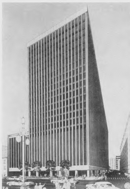
This is artist's sketch of new 24-story Canal-LaSalle Building, which houses First National Bank of Commerce's Canal-LaSalle Branch in New Orleans. Structure is joint venture of bank and Northwestern Mutual Life Insurance Co.
