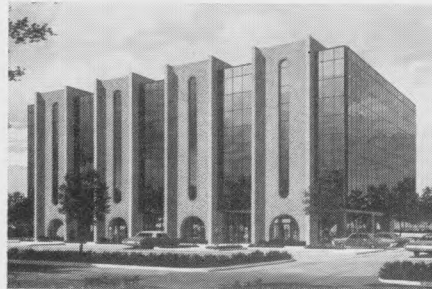
Dallas County State, Carrollton, recently opened a new building of light brown sandy-faced brick and reflective solar bronze glass.
