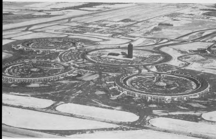
LEFT: Air photo of Kansas City International Airport centers on terminal complex of 5,000-acre facility. This new $250-million airport opened November 11, 1972. Initial development called for three circular terminal buildings with combined capacity for handling 10-12 million passengers per year. Fourth module will be added when needed. Reading counter-clockwise, Braniff and Frontier are located in Terminal "A"; TWA and Delta in Terminal "B" and Continental,
