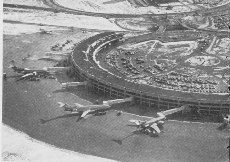
United, North Central and Ozark in Terminal "C." Mexicana Airlines will begin nonstop service from Mexico this year and will operate from Terminal "C." RIGHT: Close-up of one of terminal buildings shows parked aircraft and jetway loading bridges on apron or air side of building. Terminal loop roads and auto parking facilities are shown on passenger access or ground side of structure.
