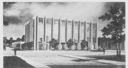
First City Bank, Hopkinsville, has broken ground for a new four-story, 40,000-square-foot building. The structure, to cost more than $1.7 million, is expected to be completed by mid-1974.
