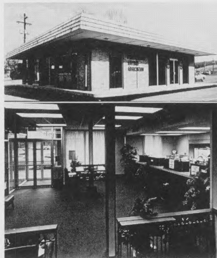
TOP: Attractive exterior of Central Pennsylvania Savings four-section modular building.
