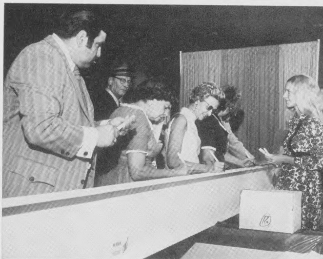
LEFT—Some 4,000 Tulsans accepted the invitation of First National to "get on the beam" and sign the 22-foot topping out I-beam that was displayed in the bank's lobby for three days recently. The beam, when hoisted into place atop the bank's new 41-story tower, completed the structural work on the building, which is the state's tallest.
