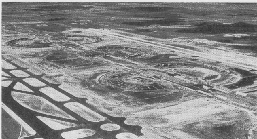
Construction of Dallas/Ft. Worth Airport has reached this stage. Outline of terminal half loops can be distinguished.
