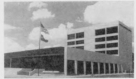
First National, Conroe, recently opened its new $2.5-million, six-floor bank and office building. The structure's exterior is textured beige concrete with large smoked glass areas.
