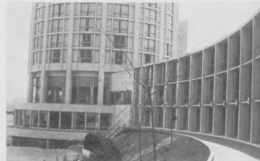
Lobby of Stouffer's (wide glassed area in rear) faces riverfront. In addition to rooms in circular building, Stouffer's has additional rooms in three-story structures attached to each side.
