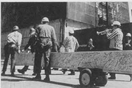
Dixieland band accompanies workers and beam.
