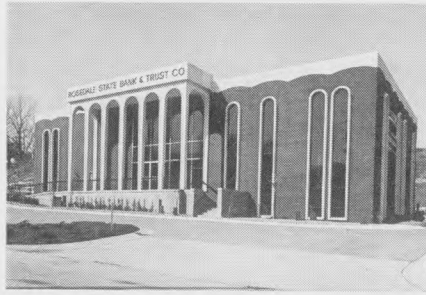
Rosedale State, Kansas City, Kan., purchased land for its new building from the Urban Renewal Agency in 1969. The bank building is located in the University-Rosedale urban renewal project.
