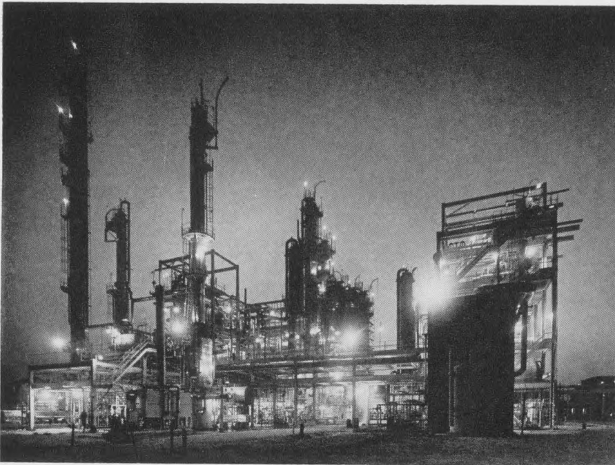
Georgia-Pacific's new $44-million Plaquemine, La., chemical complex will produce 100 million gallons of methanol annually, using new low-pressure process, plus 200 million pounds of phenol and 120 million pounds of acetone. Large part of production will supply raw materials for G-P plants that make adhesives for its plywood, particleboard and hardboard plants and other special uses.
