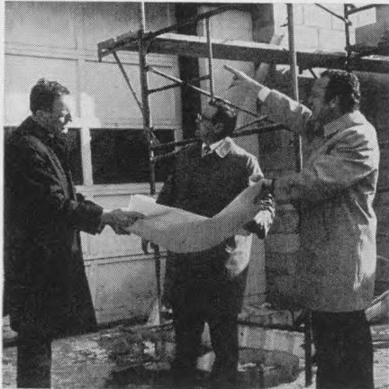
TOP: Two engineers from St. Joseph Valley Bank of Elkhart's insurance division discuss fire door size at a client's new building addition. L. to r. are Bob Rogers, safety and loss-prevention engineer; Les Shurgott, fire and rate engineer; and DeFoe Greenawalt, technical director, C & G Corp., manufacturers of Baron Mobile Homes.
