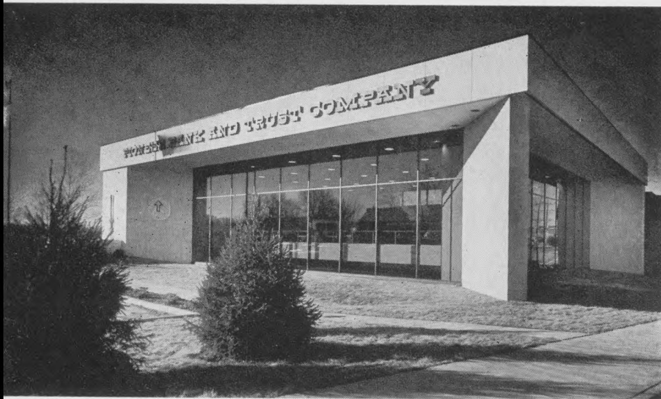
EXTERIOR of Pioneer Bank's new building features travertine marble with areas of solar bronze glass.
