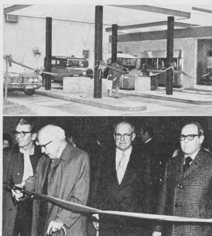
TOP: Union State's new motor bank facility has two drive-in windows and one walk-up window. BOTTOM: Participating in ribbon-cutting ceremony are: (from l.) Bob Holliday, construction superintendent, Bank Building Corp. of America, St. Louis; Lloyd E. Alquist, ch.; Glen V. Dittmar, dir.; and Chester W. Oberg, pres.
