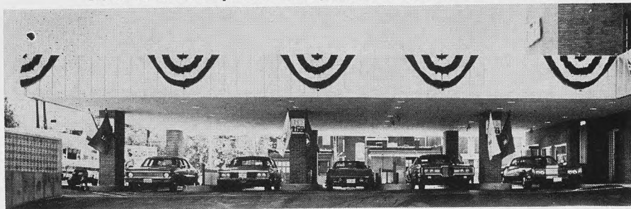
Banners decorate new drive-up installation at Tower Grove Bank, St. Louis, during grand opening celebration recently. Modernization project included five new drive-up stalls featuring a pneumatic tube system as well as two new walk-up windows. Further construction will add a four-story addition to the main building.
