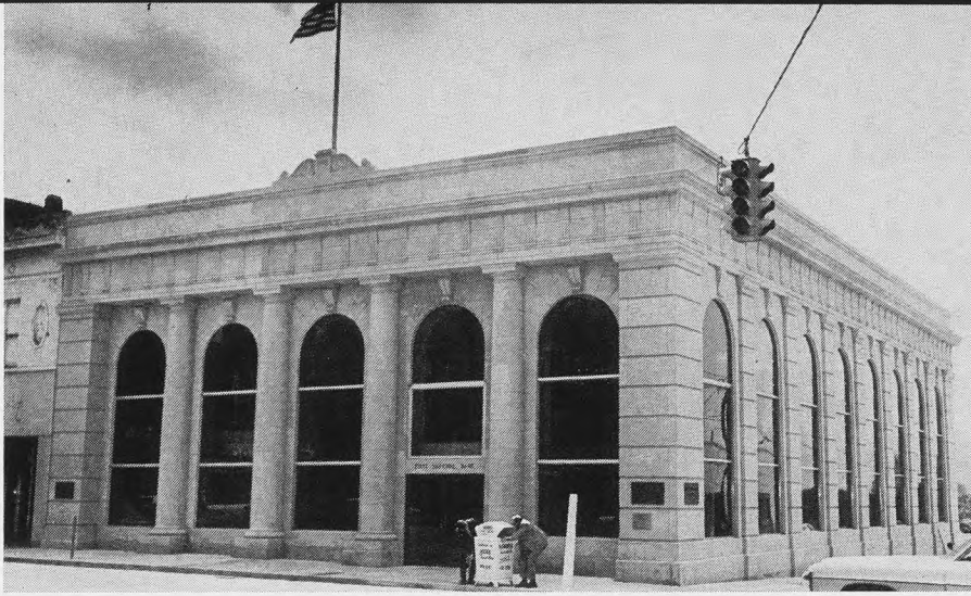
First National, McMinnville, Tenn., extended facade to left to incorporate adjacent building and almost double space.
