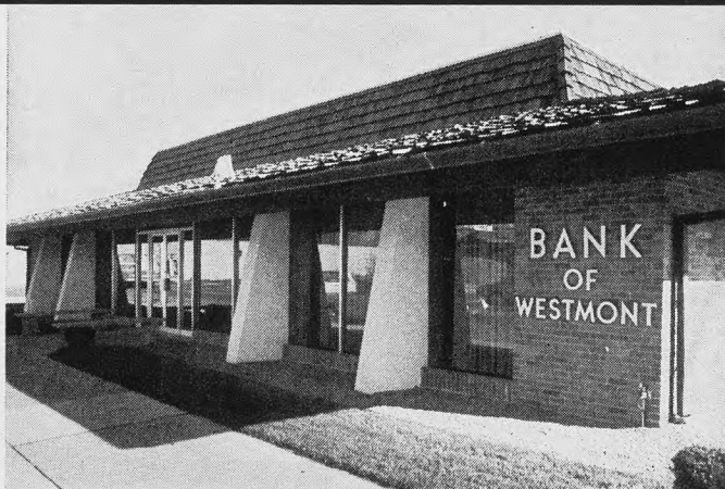
v.p., procurement; Andrew Stefik, v.p., banking services. RIGHT: One of banks using First Ogden services is Bank of Westmont. Client-banks are located in 50-mile radius of Chicago.
