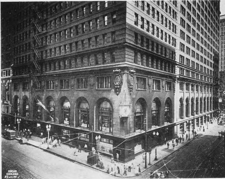
AS IT WAS—Old First Nat'l of Chicago building, city landmark for 67 years (shown here in 1953 photo), is now down to ground level in demolition. Bank's new First National Plaza will replace old structure and is scheduled for completion in 1972.
