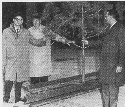
Arkansas First National, Hot Springs, recently held a topping-out ceremony to observe completion of the framework of its new bank building. Officials of the bank chose a short-leaf yellow pine tree to be used in the ceremony. From left are: W. B. Denton, exec. v.p.; Thomas W. Stone, ch. and chief exec. off.; and L. E. Powell, v.p. and cash.
