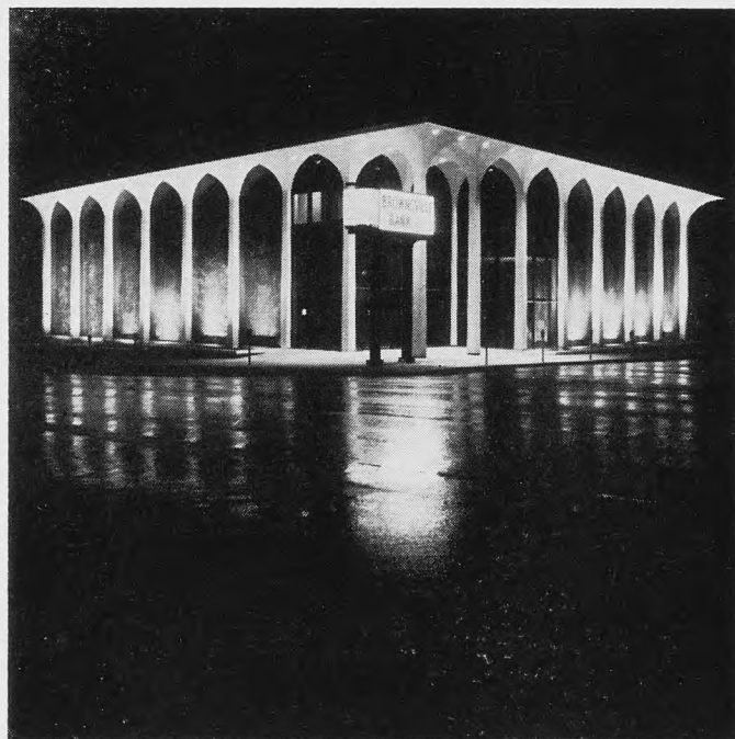
Facade of new Brownsville Bank building gleams at night.
