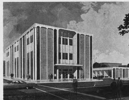
Exterior of Second National building features pre-cast concrete, brick and panels of granite and aluminum.
