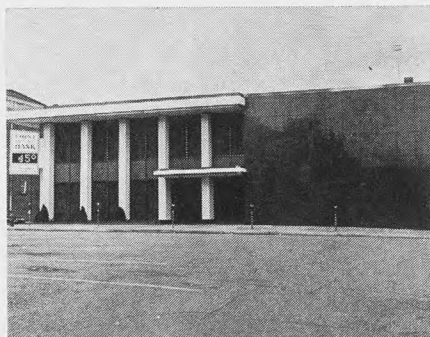
Exterior of new home of First of West Plains is made of dark green granite, with white marble exposed aggregate columns and porcelain enamel facings.
