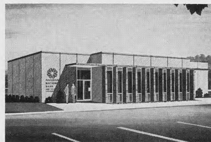
American National's new Lee Highway Branch building will be made of pre-cast brick panels in a herringbone pattern with slate columns. The 3,200-square-foot facility will have two drive-in windows.
