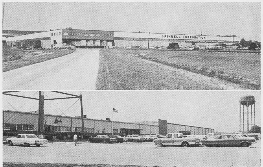
Grinnell Corp. (top) was first major industry to move to Princeton at urging of bankers Williams and Lamb. Plant employs 300. Arvin Industries (bottom) employs 1,700 from Princeton area; manufactures radio and stereo components. Water tower at far right stands on 52-acre industrial tract where construction has begun on a new $5 million plant for Federal-Mogul Corp.
