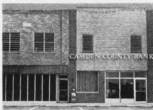
CAMDEN COUNTY BANK CAMDENTON, MO. FEBRUARY 1, 1968
