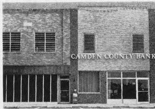
CAMDEN COUNTY BANK CAMDENTON, MO. FEBRUARY 1, 1968
