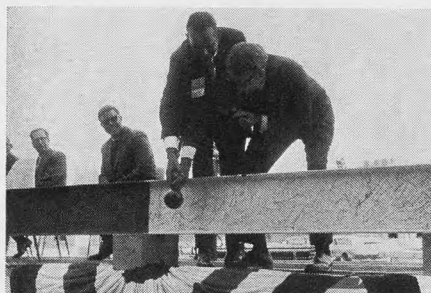
J. W. McLean (l.) Liberty National pres., and H. T. Griffin, head of H. T. Griffin Enterprises, owner of the Liberty Bank Tower, break a vial of "black gold" on the topping-out beam of the new building.
