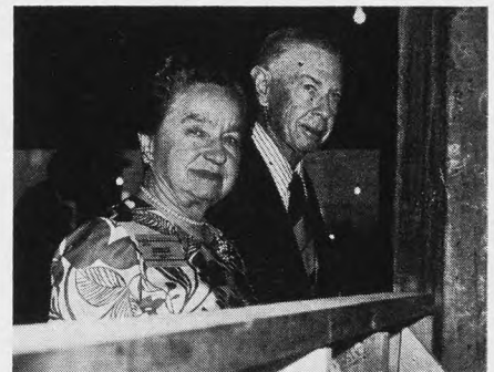
Liberty National's chairman and his wife, Mr. and Mrs. Harvey P. Everest, view downtown Oklahoma City through the steel skeleton of the rising Liberty National Tower. The bank held a cocktail party so Oklahoma Bankers Association members could inspect construction progress of the tower, which will reach 35 stories and reportedly will be Oklahoma City's tallest building. The "construction atmosphere" of the party was accented by bankers wearing imitation steel helmets made of cellophane. A "topping-out" ceremony to mark completion of the steel structure is planned for later this month.
