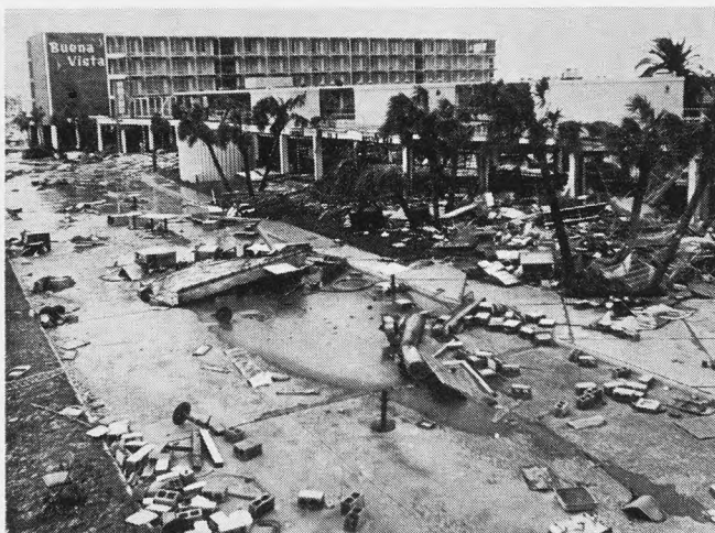
LEFT: Camille was no lady because what lady would leave debris like this lying around home of her host? RIGHT: When members of Missis-
