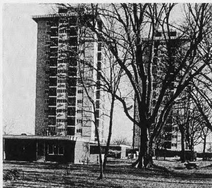
Housing complex, located in Poplar Bluff, was built by Butler & Associates, Springfield, recipient of First Missouri Development Finance Corp. loan.
