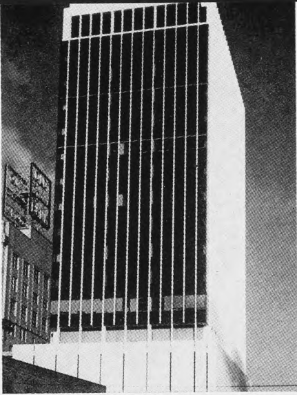
Evansville skyline is now dominated by Old National's new tower. At left is former bank quarters, being razed for completion of the tower complex.
