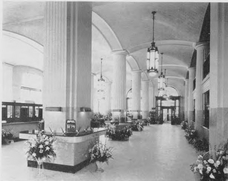
View of the enlarged and remodeled lobby of the Union Planters National Bank and Trust Company, Memphis, Tennessee.
