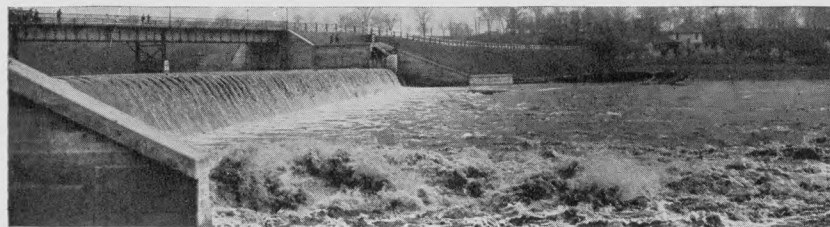
View of the Dam at Lake Decatur, Decatur, Illinois.
