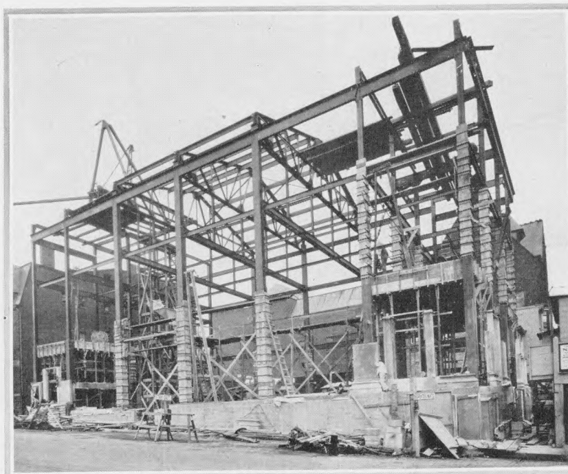
The Newburgh Savings Bank, Newburgh, New York. Steel trusses span the width of the building and give a 60 by 14 feet floor space free of columns.
