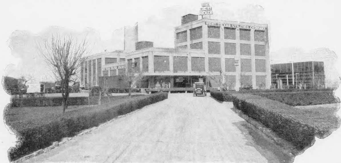
A typical, modern ice plant which serves a Texas city of over 16,000 population and provides ice for retail stations serving a considerable rural territory
