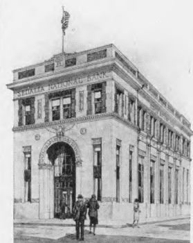
SEDALIA NATIONAL BANK SEDALIA, MISSOURI 27 ft. wide and 91 ft. deep, 2 stories, to be completed December, 1928.
