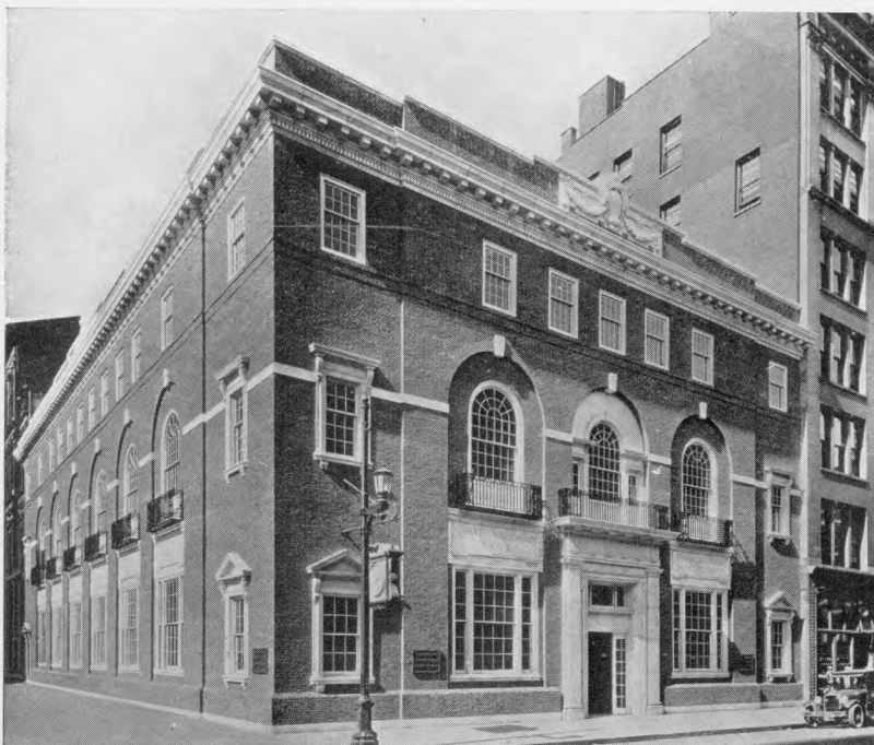
Fifth Street and Court Place exterior of the new home of the First National Bank and Kentucky Title Trust Company, Louisville.
