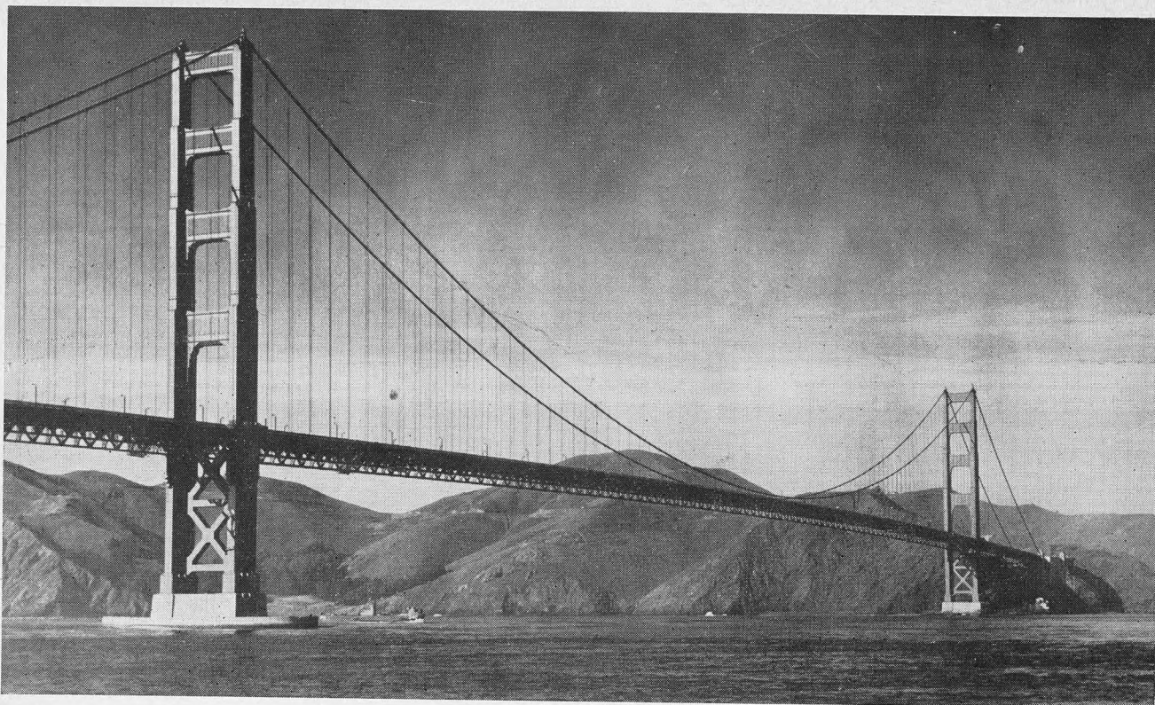
A TOTAL of 16 holes, ranging in depth from 15 to 141 feet, was drilled in 90 days by Longyear crews locating piers and anchorage sites for the Golden Gate bridge at San Francisco. The work was carried out successfully during winter months under extremely severe weather conditions and highly difficult tidal conditions.
