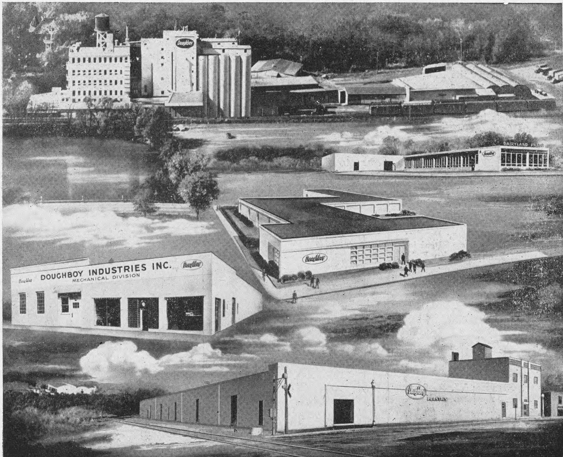
FLOUR AND FEED MILL DAIRYLAND PRESS MAIN OFFICE MECHANICAL DIVISION PLASTICS FACTORY
