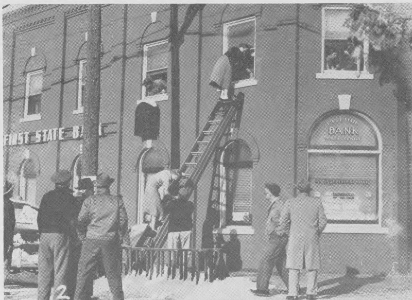
ON-THE-SCENE photograph snapped at Sauk Centre's First State Bank fire.
