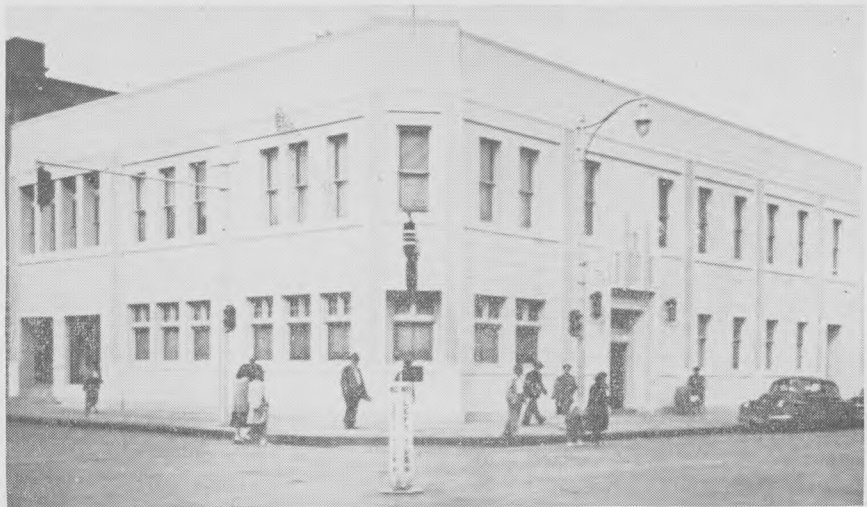
Here is the remodeled and enlarged building of the Security Trust & Savings Bank, Billings, which celebrated its 33rd anniversary Oct. 10.
