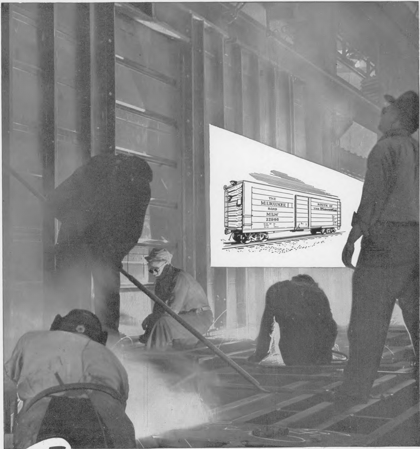
Welding side on all-steel, plywood-lined box car
