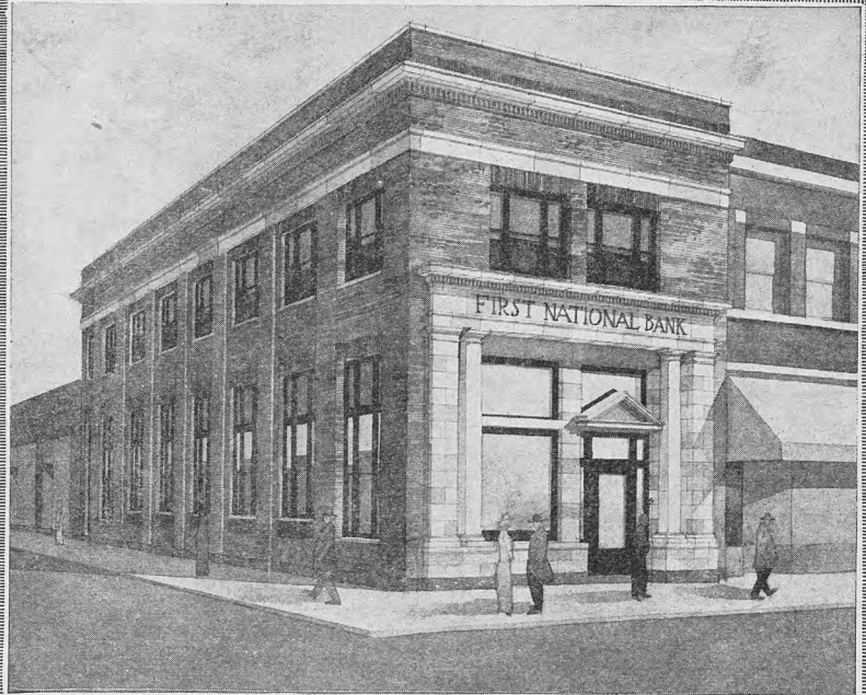
FIRST NATIONAL BANK, PARK RAPIDS, MINNESOTA (Under Construction)
