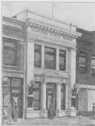
NEW SCANDIA STATE BANK BUILDING, FERGUS FALLS, MINN.
