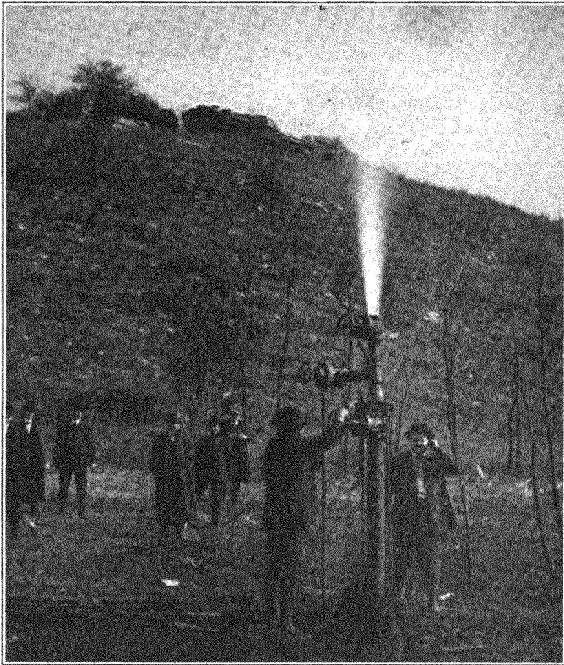
GAS WELL PRODUCING 20,000 FEET PER DAY.
