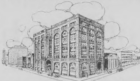
BANK OF COMMERCE BUILDING First. Ave South and Fourth St.
