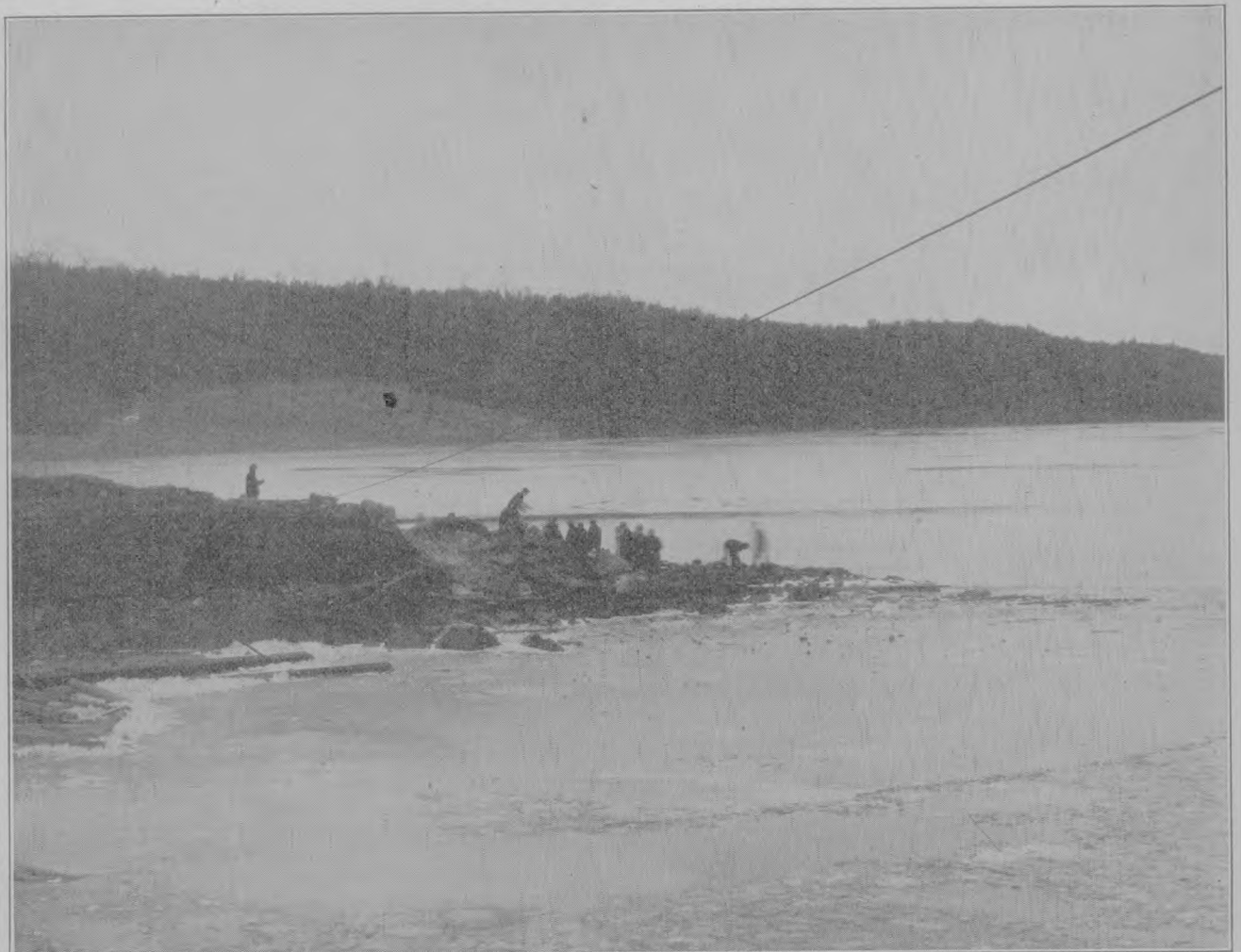
EXCAVATION FOR LOG SLUICING ABOVE BEAR TRAP.
