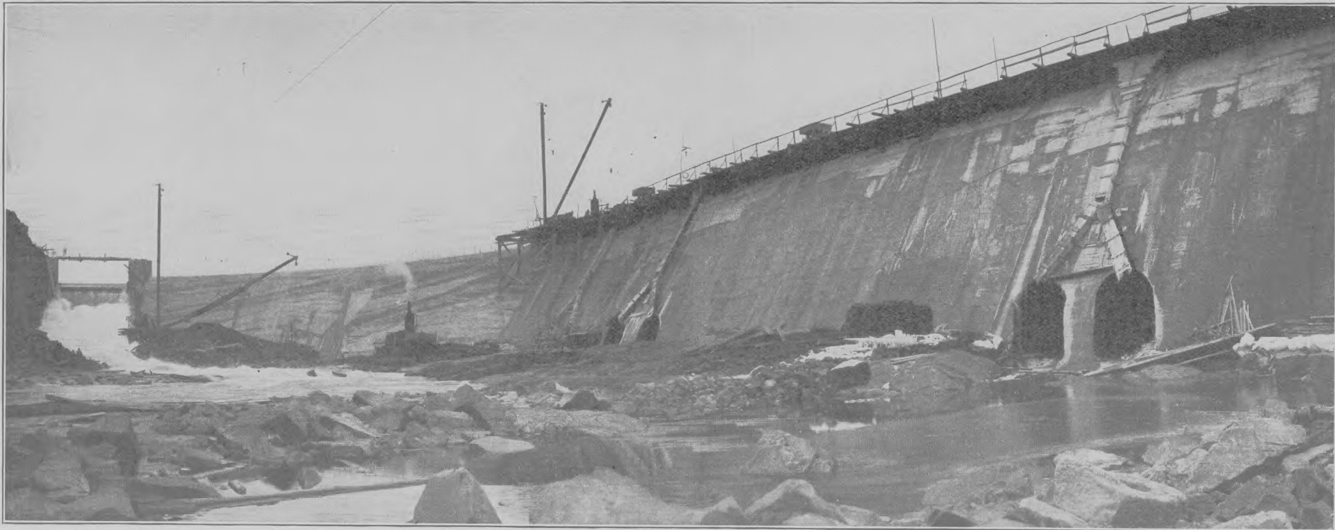
COMPLETED DAM AND LOG SLUICE OF THE MINNEAPOLIS GENERAL ELECTRIC COMPANY'S POWER PLANT AT ST. CROIX FALLS.
