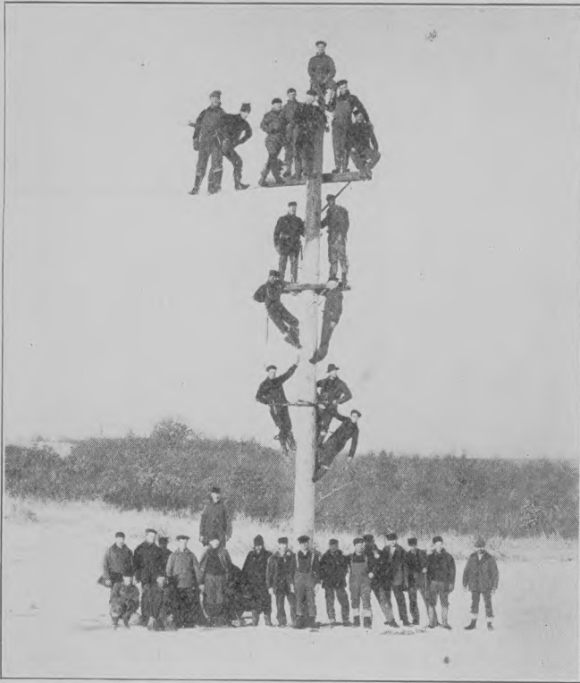
LINEMEN COMPLETING LAST SPAN TRANSMISSION LINE BETWEEN MINNEAPOLIS AND TAYLORS FALLS.
