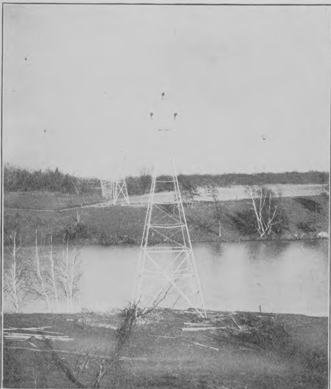
TRANSMISSION LINE LOOKING EAST ACROSS LONG LAKE.
