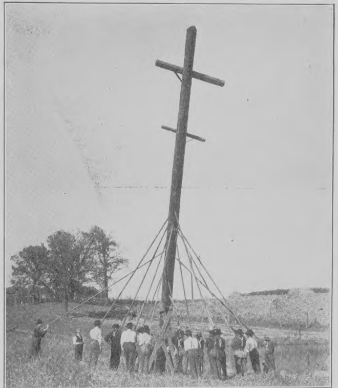
POLE CREW PIKEING 65-FOOT POLE.
