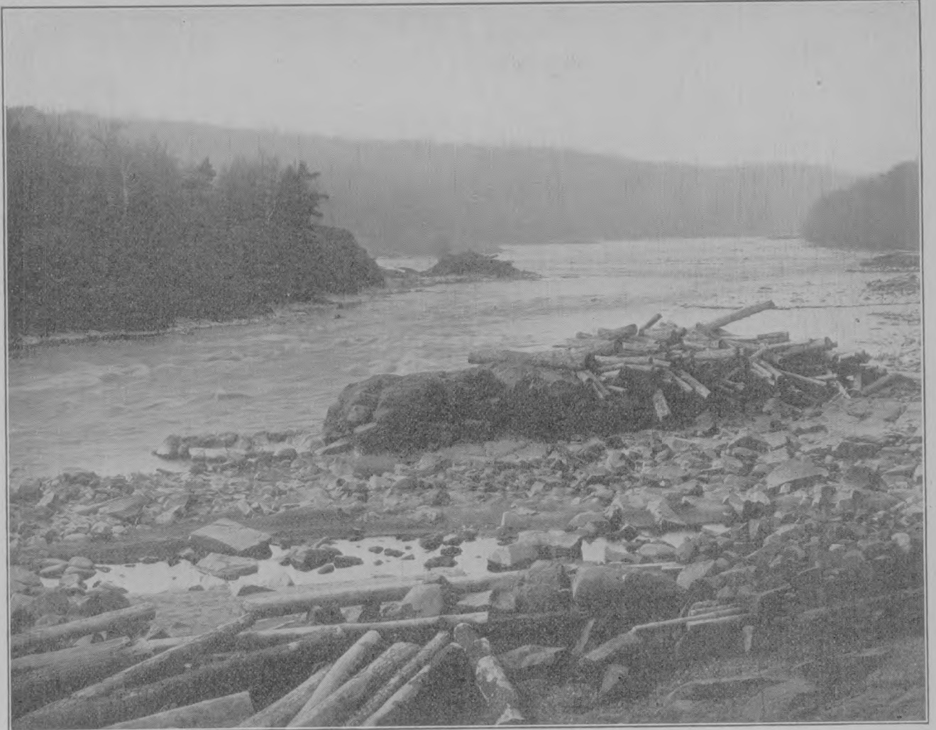
DAM SITE LOOKING UPSTREAM PREVIOUS TO BEGINNING CONSTRUCTION WORK.
