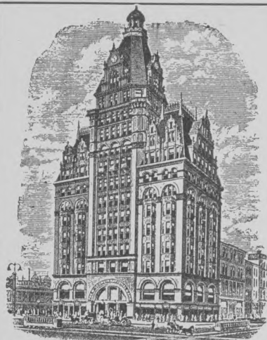
BUILDING OWNED BY THE BANK
