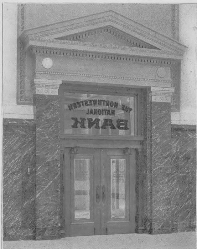
BANK ENTRANCE, FROM THE INTERIOR.
