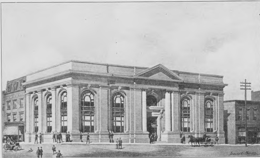
NEW BUILDING FOR THE NATIONAL BANK OF ST. JOSEPH, ST. JOSEPH, MO., IN COURSE OF ERECTION.
