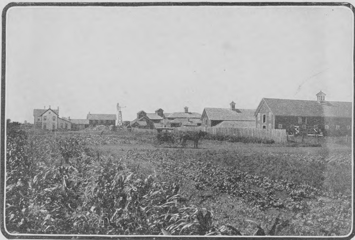
TYPICAL NORTH DAKOTA FARM BUILDINGS ON THE GREAT NORTHERN ROAD.
