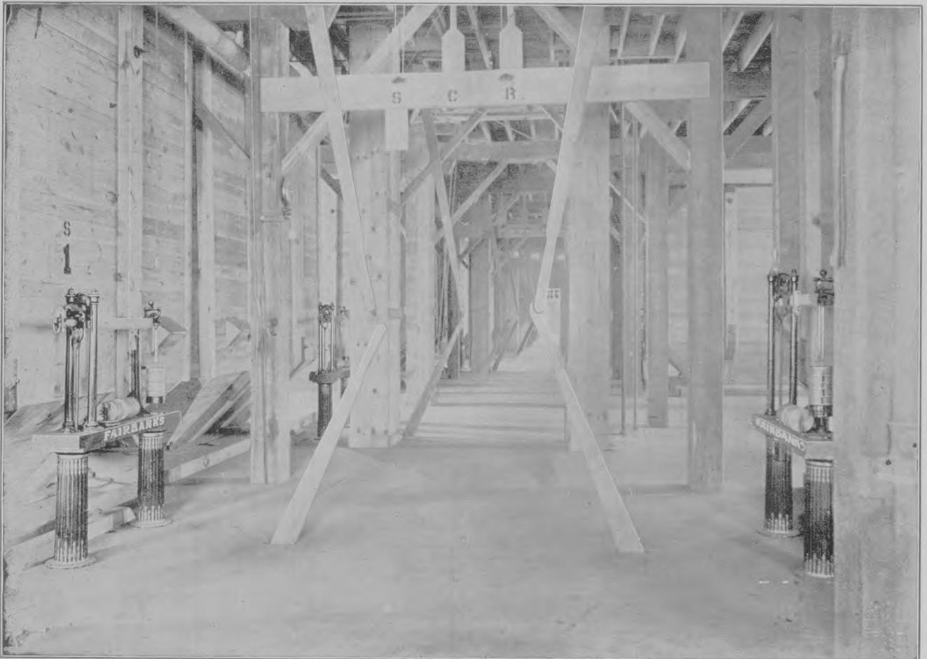
TEN FOURTEEN-HUNDRED-BUSHEL AND FIVE SIXTEEN-HHUNDRED-BUSHEL FAIRBANKS' IMPROVED HOPPER SCALES INSTALLED IN PEAVEY DULUTH TERMINAL ELEVATOR, DULUTH.
