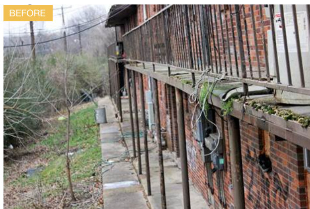
Tillman Crossing apartment complex, before and after rehabilitation
