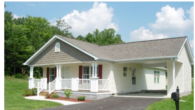
FIGURE 4: ENERGY STAR manufactured home in Morehead, Ky., developed by Frontier Housing, a Next Step Network member. Source: Next Step.
