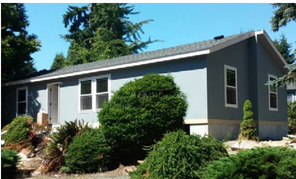
FIGURE 2: High-performance manufactured home prototype in Bothell, Wash., developed by Community Frameworks, a Next Step Network member, in partnership with Habitat for Humanity—King County. Source: Habitat for Humanity.
