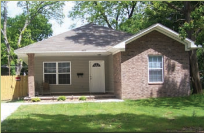
This house in the Argenta District of North Little Rock was built using green technologies. It is part of an affordable housing development undertaken by the Argenta Community Development Corp. in partnership with the Arkansas Chapter of the U.S. Green Building Council.
