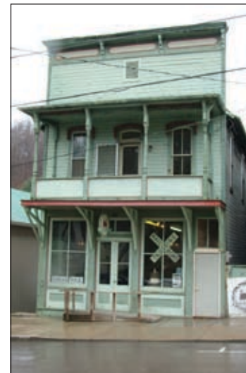
One of the buildings that is part of the New Straitsville Downtown Revitalization project in southern Ohio's Hocking Valley Coal Region.
