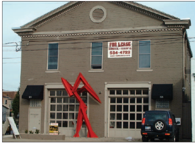
Hook and Ladder #2, one of the first firehouses in downtown Louisville, was converted into three loft-style apartments, with an art gallery on the first floor. The Downtown Housing Fund provided a 10-year, $45,000 second mortgage with an 8.5 percent interest rate.
