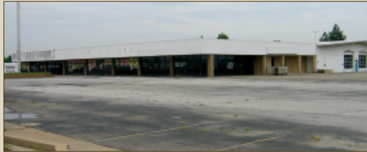
This old auto dealership in West Memphis, Ark., will be turned into the Delta Regional Transportation Technology Center next year, thanks in part to the Delta Regional Authority.
